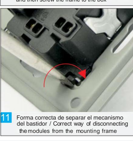
11 Forma correcta de separar el mecanismo del bastidor / Correct way of disconnecting the modules from the mounting frame
